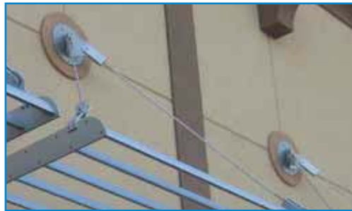
Turnbuckle Assembly
