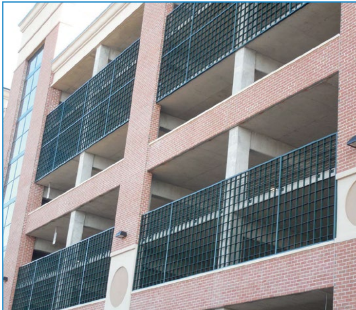
Metro Centre Parking Garage, Owings Mills, MD
