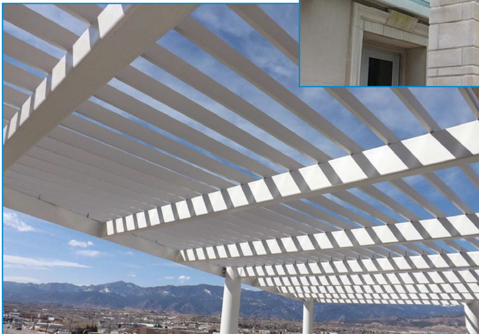
UCCS Lane Center, Colorado Springs, Colorado
