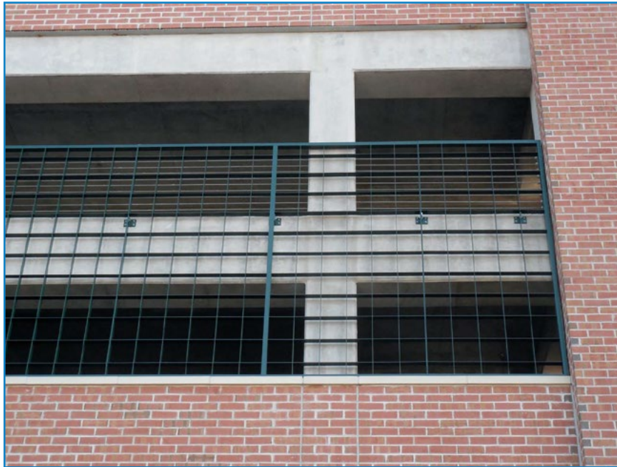
Metro Centre Parking Garage, Owings Mills, MD
