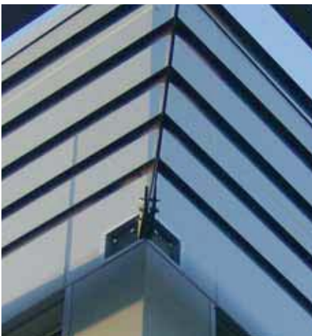
Turnbuckle Assembly
