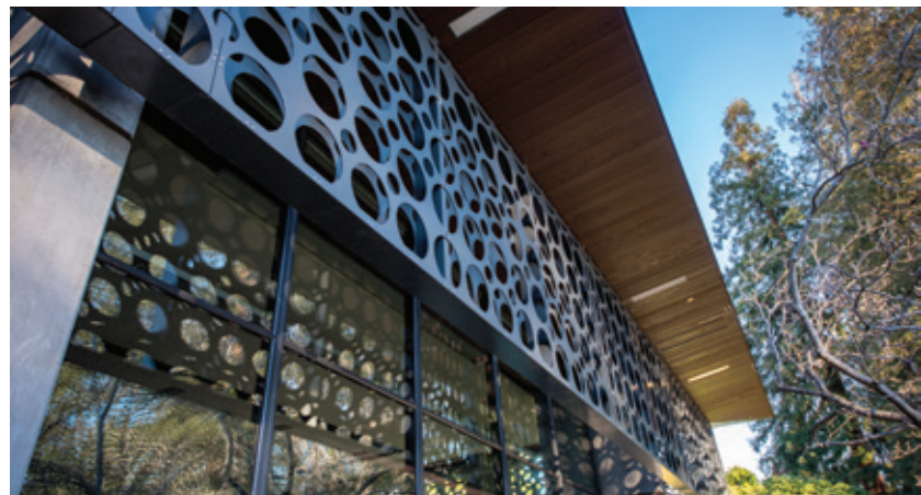
Rinconada Library Palo Alto, CA Perforated panel sunshade
