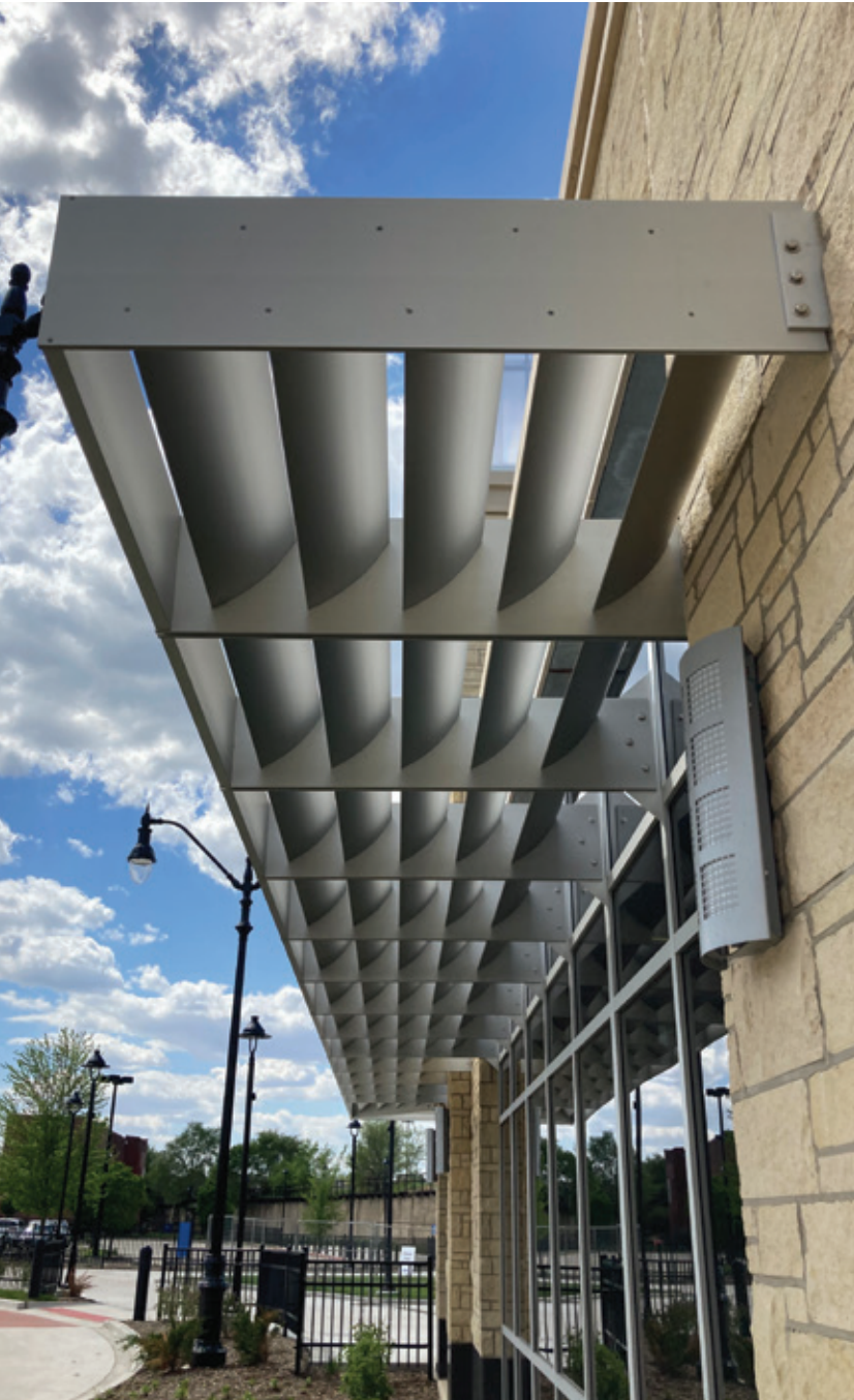
Joliet Bus Station Joliet, IL Wexford sunshades
