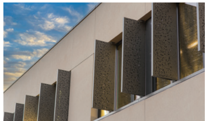
Marin Academy San Rafael, CA Perforated panel vertical sunshade
