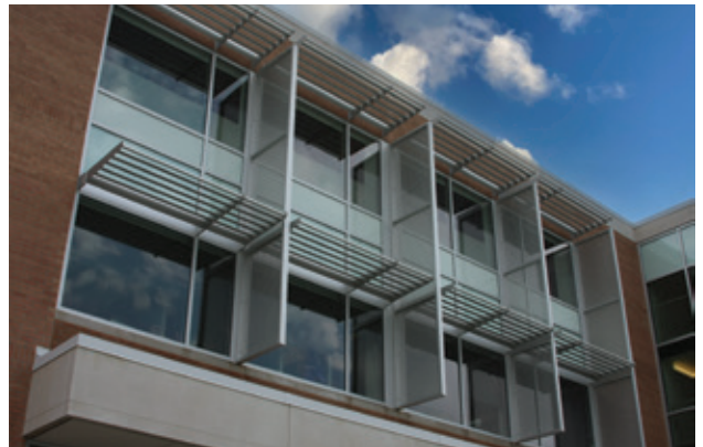
Lincoln Lancaster County Health Department Lincoln, NE Horizontal sunshades & vertical perforated panels
