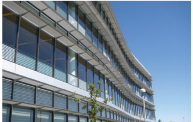
Denver Children's Hospital Denver, CO Taurus perforated panel sunshades
