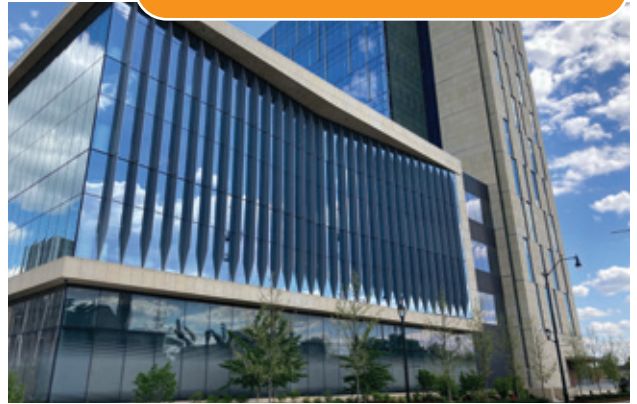
Will County Courthouse Joliet, IL Toronto vertical fins
