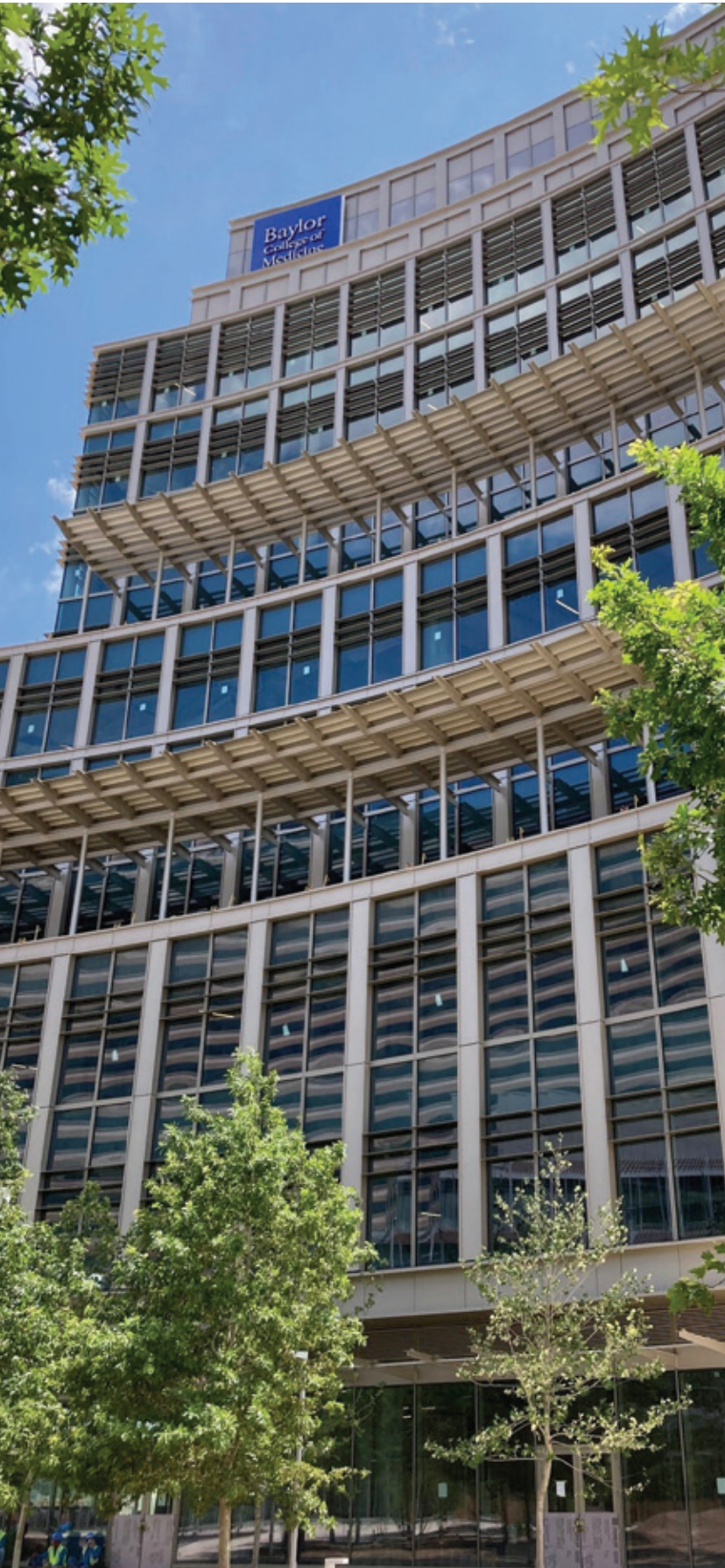
Texas Medical Center Houston, TX Custom arched blade trellises
