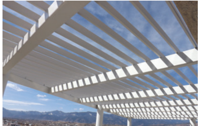
UCCS Lane Center Colorado Springs, CO Aluminum trellis
