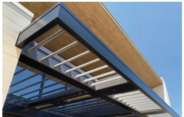
California Residence, CA Aluminum trellis
